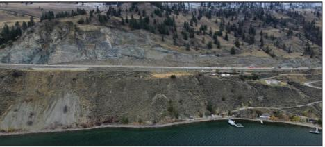
ed reinforcement. Additional rock anchors will also be installed to secure the slope, followed by repairs to the road's surface and drainage improvements.
